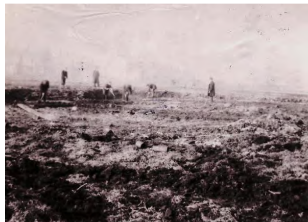
Fig. 19. Clearing a stream on Hale Moss (HEB)
