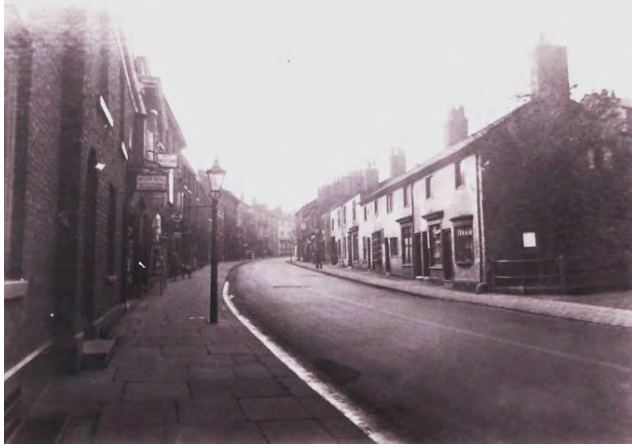
Fig. 31. Later view of northern end of Church Street (HEB)
