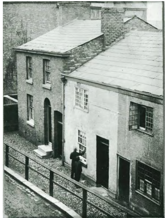
Fig. 33. Old buildings in Lower George Street (HP)
