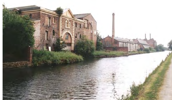
Fig. 37. The 1833 canal warehouse (DGB)
