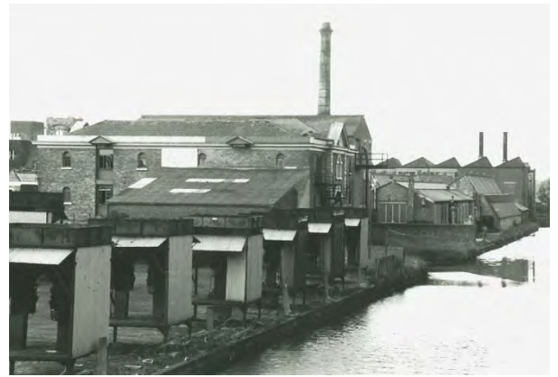
Fig. 40. Coal staithes before demolition; 1833 warehouse (Luxi Products), beyond (DGB)
