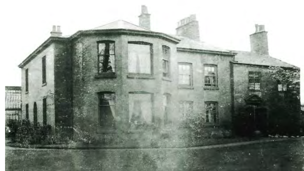
Fig. 30. Mill manager's house on Stamford Road (Grosvenor Road) (HEB)
