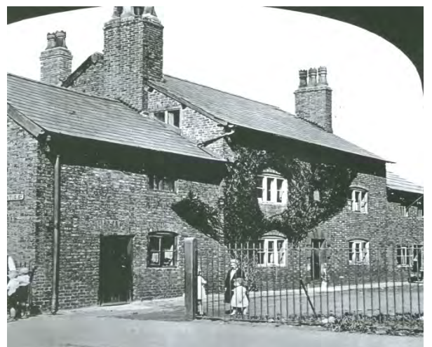
Fig. 42. Duke's Cottages, part of former workhouse before demolition (TLS)
