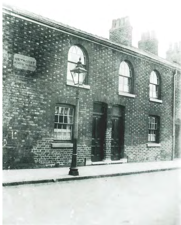
Fig. 44. Methodist Sunday school, 1858, Dale Street (HEB)
