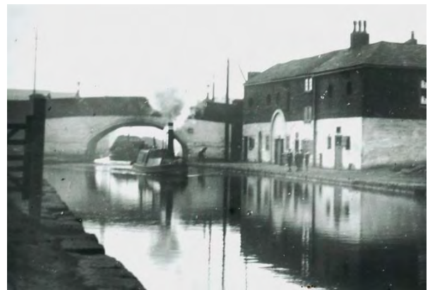
Fig. 41. Warehouses on the north side of the canal before demolition (TLS)
