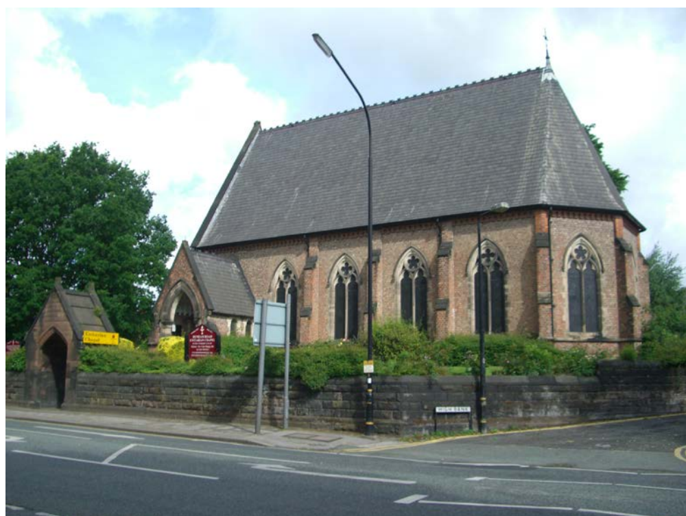
The Unitarian Chapel on the Dunham Road, Altrincham
