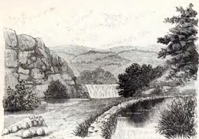
MILL DAM AND FALLS OF IRWELL.
