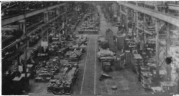
40. Richards' erection shop for medium size horizontal borers. (Company brochure, late 1940s.)
