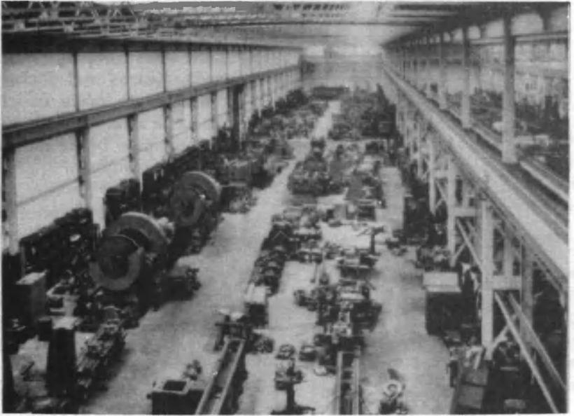
35. One of Churchill's thirteen assembly bays covering altogether 160,000 square feet.
