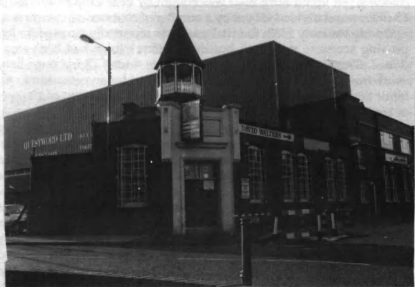
48. A corner of the H W Kearns (later Kearns-Richards) building in 1995. The huge production plant has had a modern cladding fitted.
