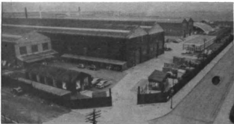
41. Tilghmans' No. 4 plant housing machine shop, compressor erection, and dust frame division.
