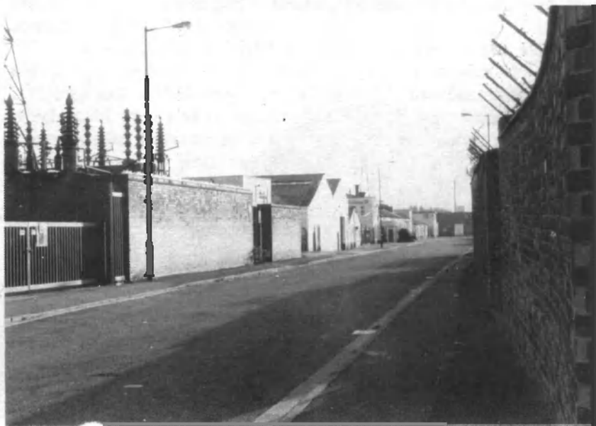
52. Davenport Lane 1995. Shows electricity sub-station on left where Altrincham Electric Supply Co. stood. P I Castings can be seen further down on left.
