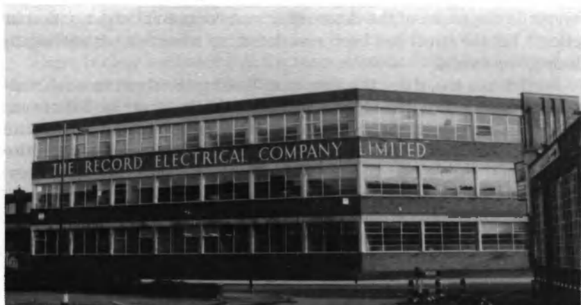
57. Record Electrical – who now occupy part of the middle floor.
