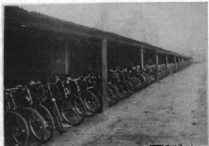
29. Record Electrical Company: bike shed, 1930s. (Company photograph.)
