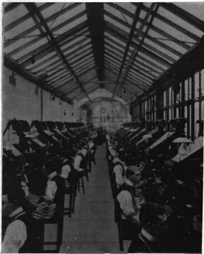
16. The Sheffield Daily Telegraph installation of twenty-seven Linotype composing machines. (From company brochure, pre-1914.)
