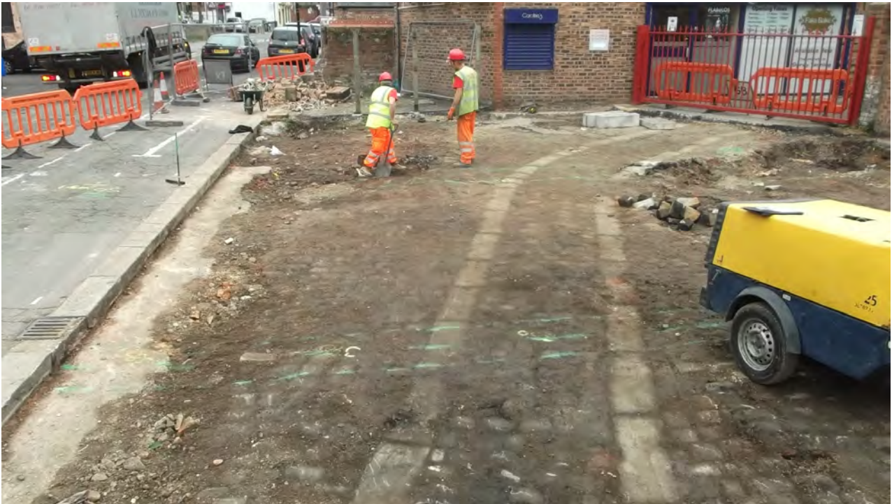
Plate 6.3 View of exposed roadway looking towards the alleyway to Greenwood St.
