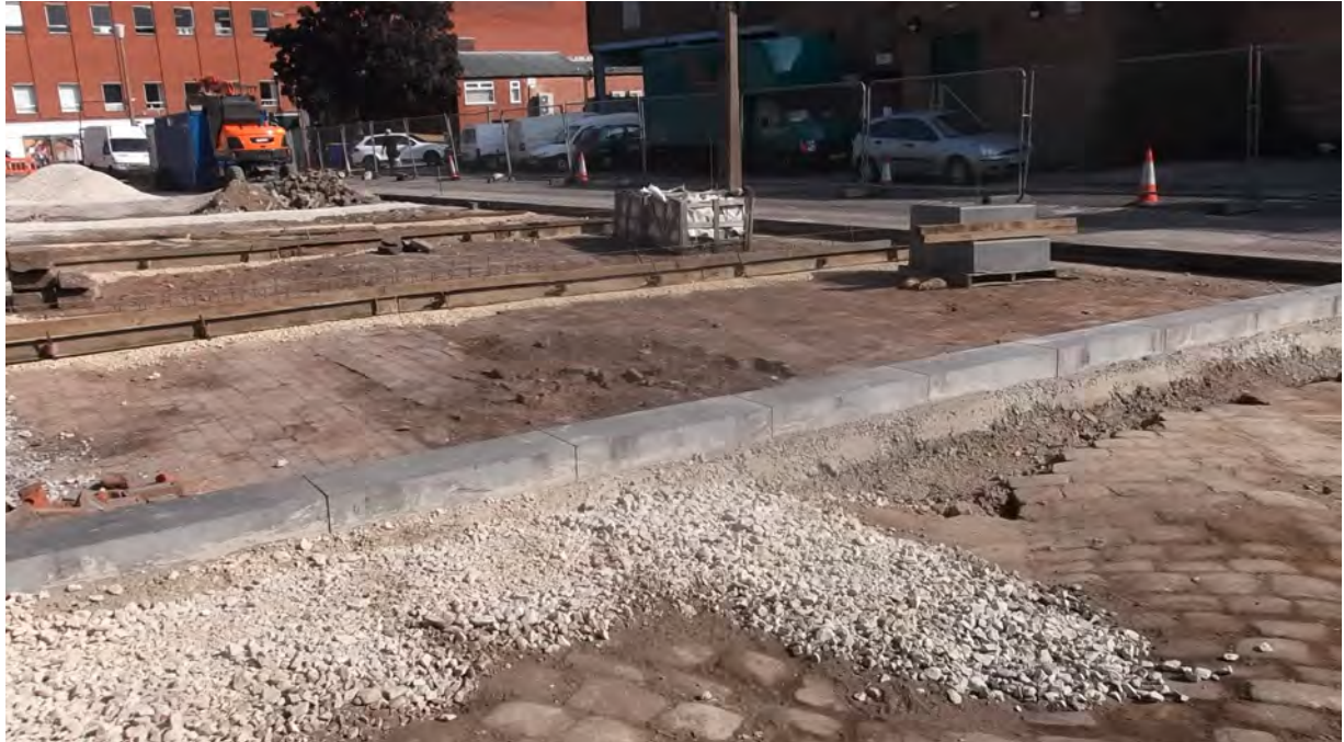
Plate 6.5 General view of drain conduits across the site to Central Way
