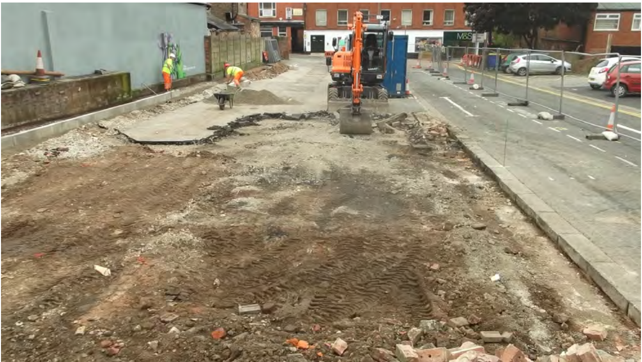
Plate 6.4 View NE towards Shaw's Road showing levels removed above the roadway.
