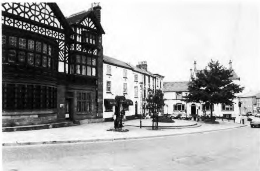
Old Market Place 1991. Refurbishment arranged by the Altrincham and Bowdon Civic Society with the cooperation of Trafford Borough Council.
