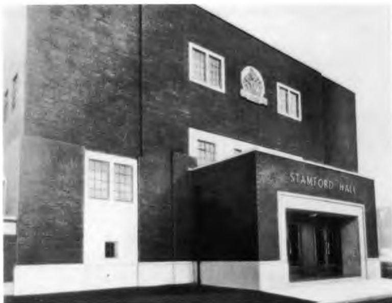
Stamford Hall Exterior 1940.
