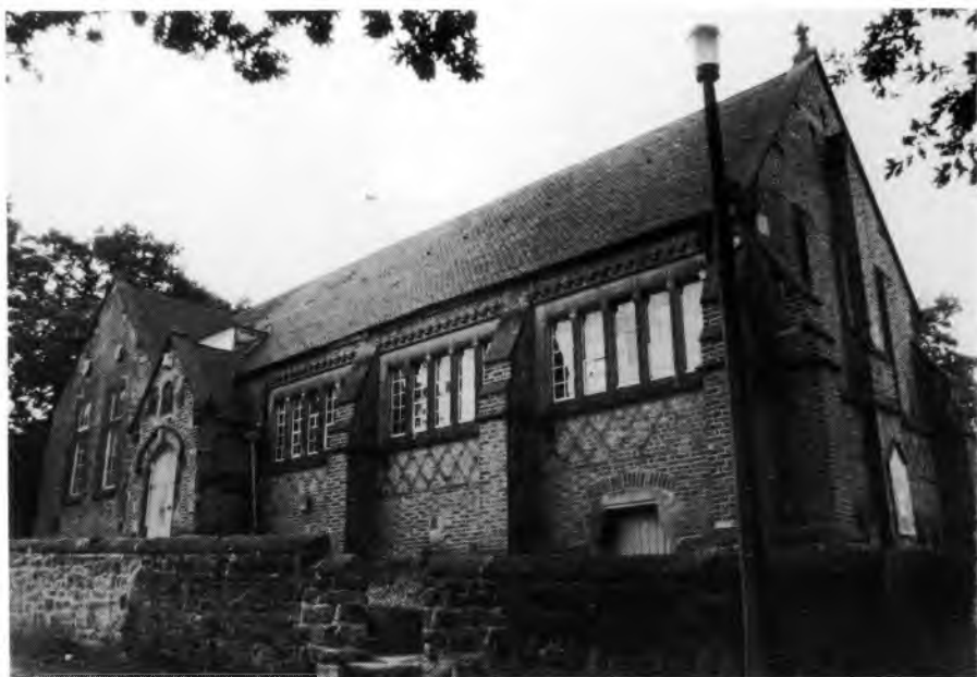
Seamons Moss School. Built in 1867; note the Gothic doorway. The school began 100 years earlier at Oldfield House nearby, not to be confused with Oldfield Hall built by the same Thomas Walton.
