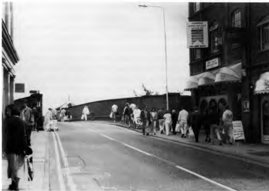
Moss Lane Bridge. No pavement on the left.
