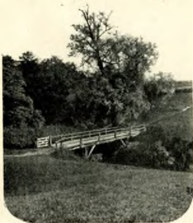
The Birken Bridge.
