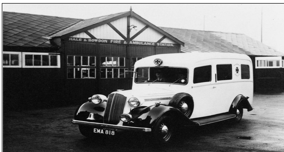
Hale Fire & Ambulance Station (1957). The site is now the small car park backing on to the railway off Cecil Road (AAIA).
