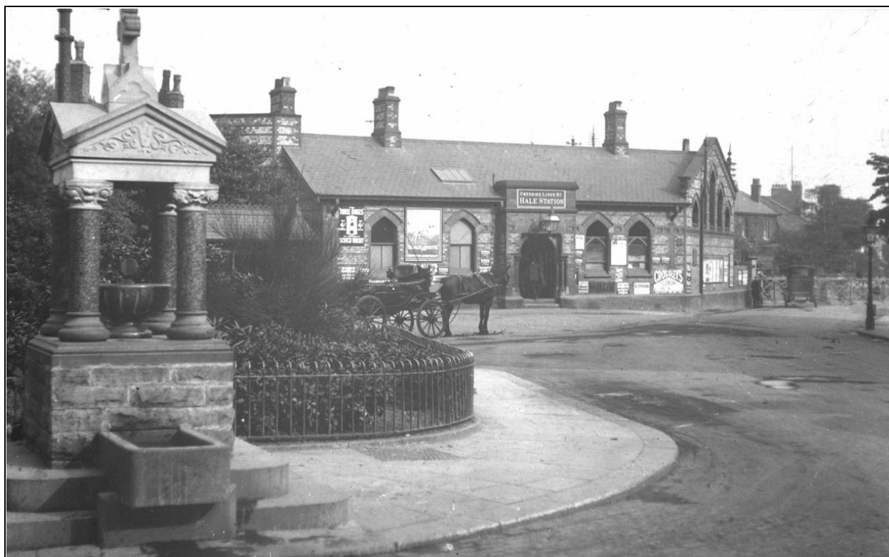
Hale Station and the 1908 George Baker Walsh memorial drinking fountain with horse trough (1920s, AAIA).
