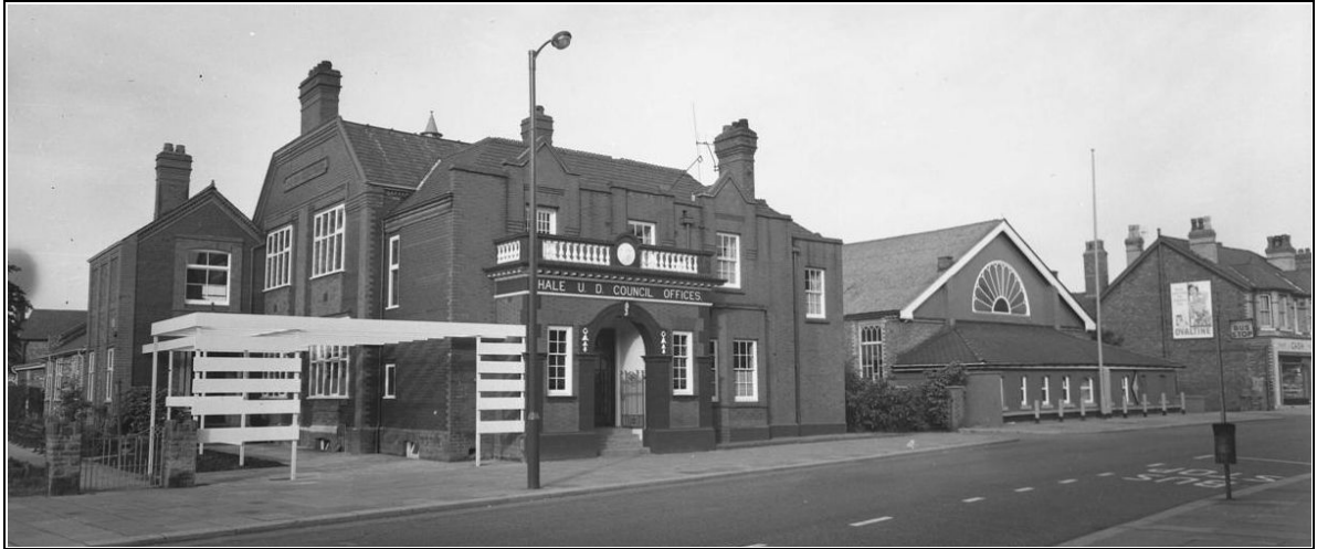
Council Offices and Drill Hall in 1963 demolished 1970. Now the site of a hotel and shops. The Bowling Green is to the left (AAIA).
