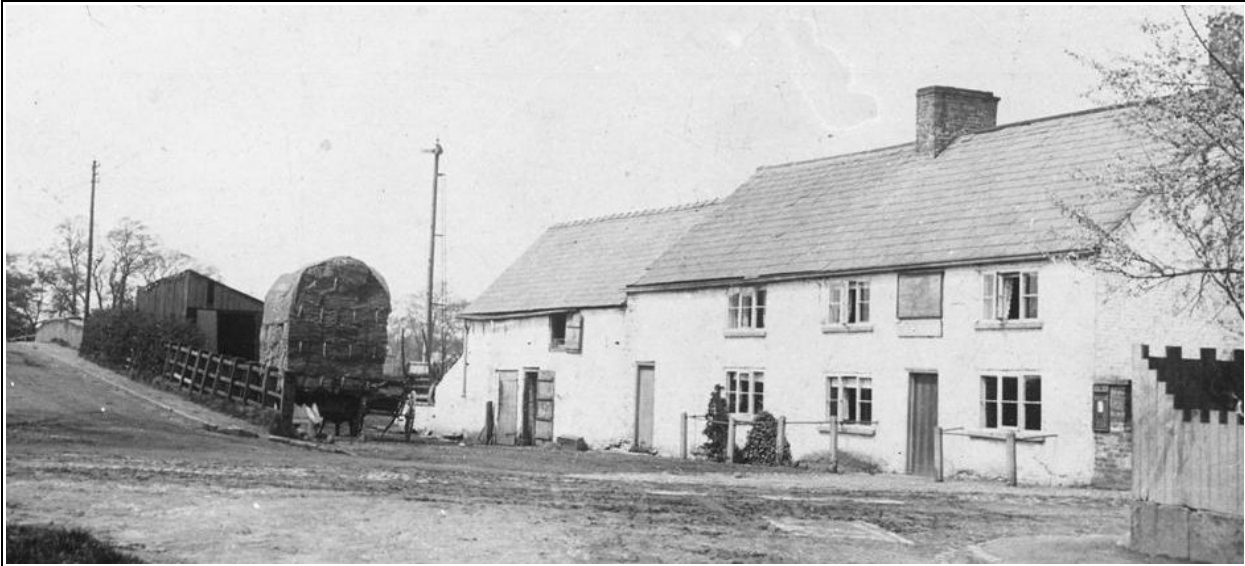
The original Bleeding Wolf Farm and Inn on the corner of Heather Road and Ashley Road demolished in 1898 (c1880, AAIA).
