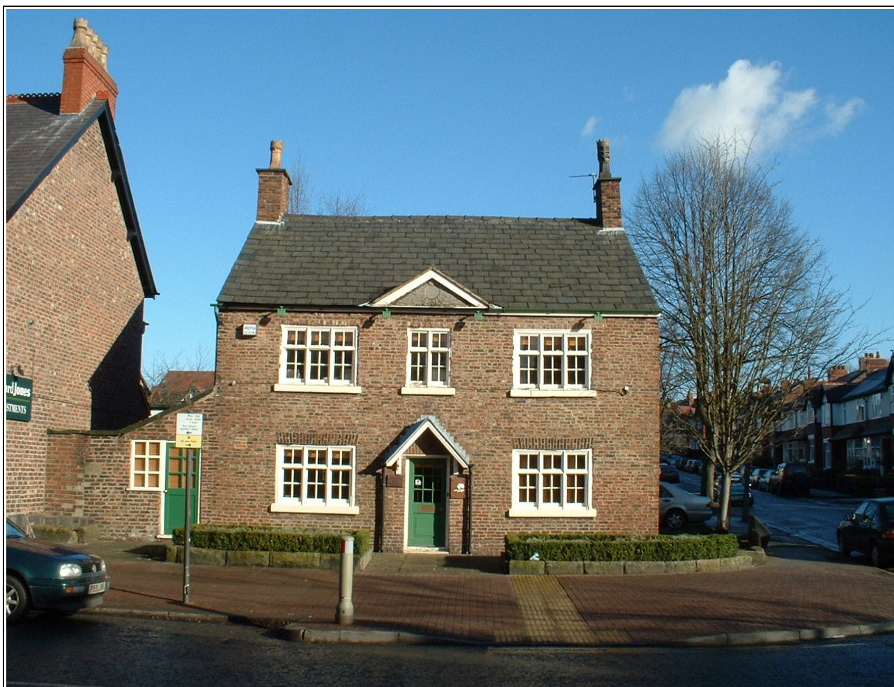
Ollerbarrow Farm at the junction of Leigh Road and Ashley Road in recent times (DM).
