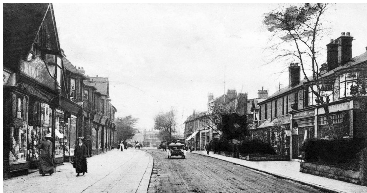
Ashley Road looking towards Hale railway station (AAIA).
