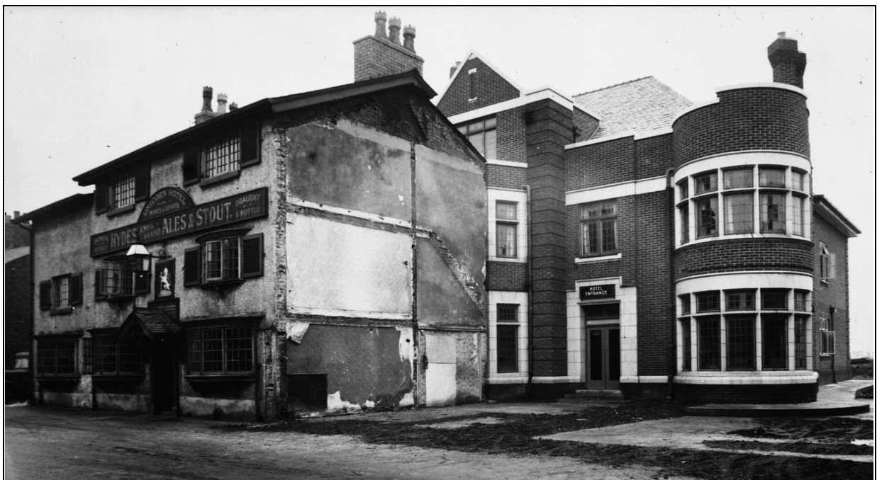
The Unicorn, Hale Barns being demolished and replaced by the building behind in 1935 (AAIA).
